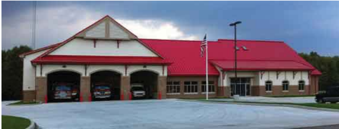
Figure 1. New Bristol Township Fire Station
