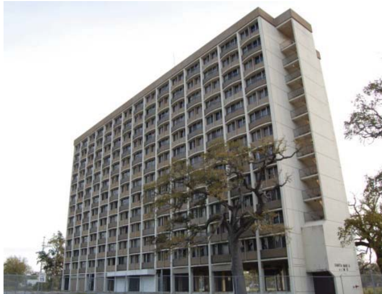
Figure 1. Santa Maria de la Mer (damaged facility)
