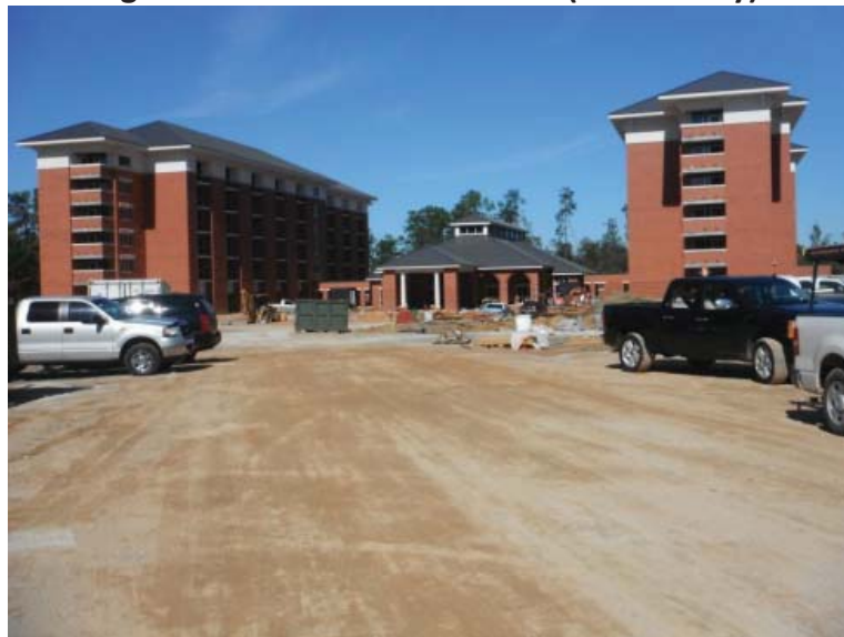
Figure 2. Santa Maria de la Mer (new facility)
