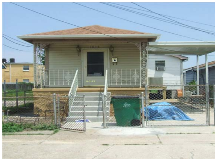
Figure 1: Elevated Home in Gretna, Louisiana Source: Louisiana OCD Applicant Tracking System
