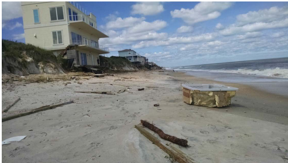
Figure 1: Damages at North Beach
